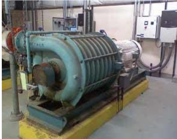
Aeration systems are the largest single user of energy at a typical wastewater treatment plant.
