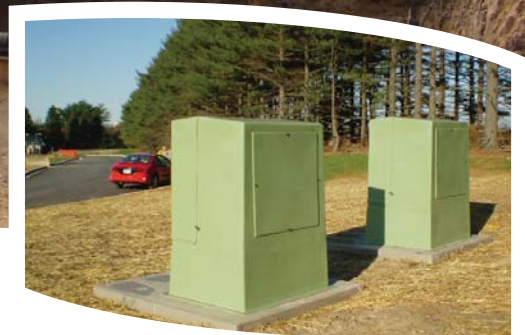
New BGE design district regulator station being installed in Linthicum, MD.
