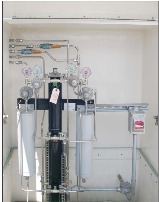
Figure 8.0 - Single PIC Installed in Becker CAB Series Fiberglass Enclosure A Becker PIC Pressure Instrumentation Column is installed inside a Becker CAB Fiberglass Cabinet. The PIC provides conditioned and regulated supply gas to four tube switching valves. The outputs to the tube switching valves are located in the upper left corner of the cabinet. The PIC includes optional dual FD-1500 Filter-Dryers complete with independent regulation systems to meet higher capacity requirements. Each FD-1500 and regulator set feeds a pair of the tube switching valves. The PIC system also includes the optional stainless steel components to comply with specific customer requirements of no brass material in the system. The catalytic face heater is hard wired with 120 V A.C. starting voltage complete with the disconnect located inside the fiberglass enclosure.
