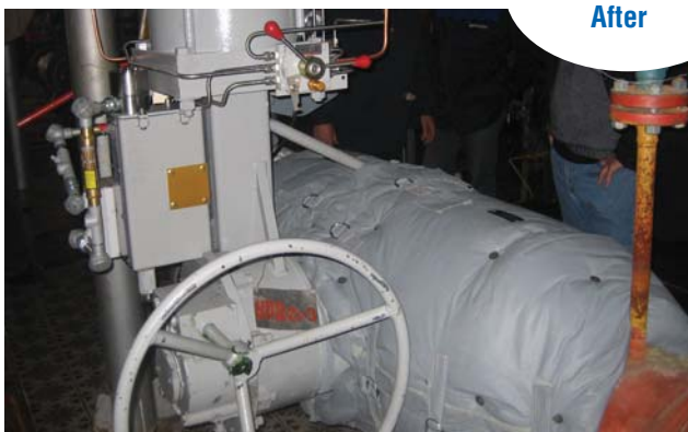
Figure 2 - Typical Becker Control Valve Installation AFTER Installing ANJ
