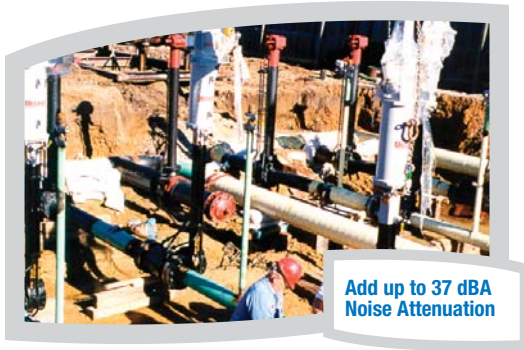
Figure 13 - Installation of Becker Below Ground Regulators (Prior to Backfill)
