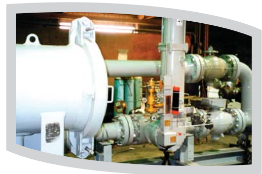
Figure 16 - Becker RPSR Actuators are ideal for Surge Control/Recycle Valves
