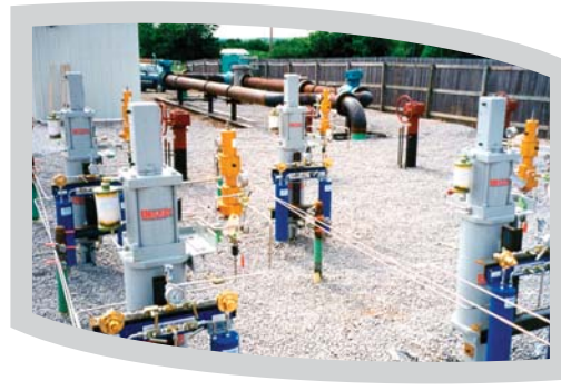
Figure 14 - Installation of Becker Below Ground Regulators (After Backfill)
