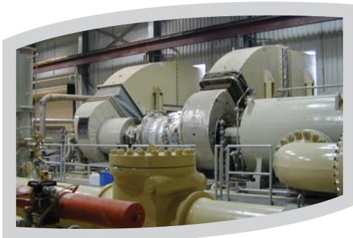
Figure 11 - Surge Control Valves Centrifugal Natural Gas Compressors (Natural Gas Transmission Industry) Becker Surge Control Valves provide increased protection for Centrifugal Natural Gas Compressors. The Surge Control Valve will open rapidly upon potential surge to protect the centrifugal compressor mechanism. Becker Surge Control Valves are well accepted by many Natural Gas Transmission companies and Natural Gas Compressor manufacturers throughout the industry. For additional information see Becker’s Surge Control Valve Brochure (SCV)..
